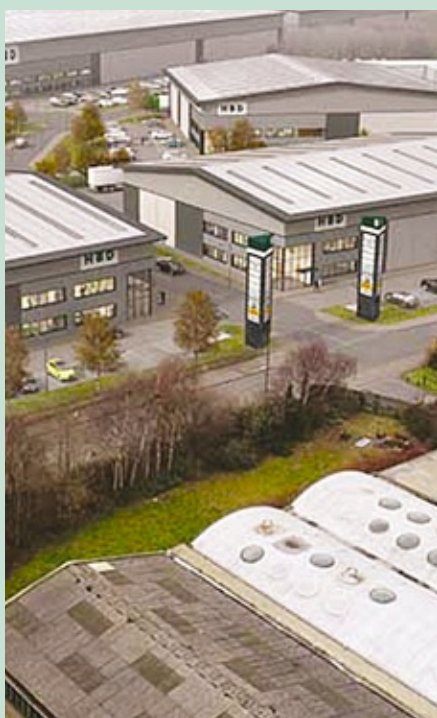
Henry Boot Development has started work to regenerate the 44-acre former James Bridge Copper Works in Walsall
